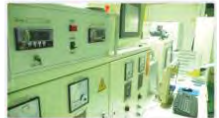
風洞實驗室 LAB OF TESTING FANS
